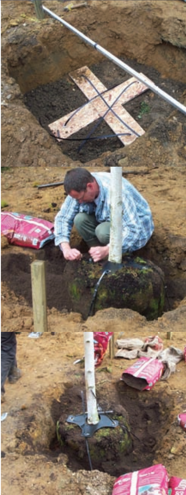
A planting involving 200 litre trees at Westonbirt Arboretum using the Arbortech Root Anchor.
